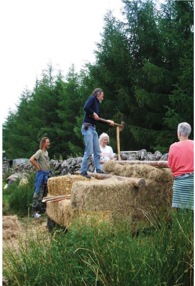
final stages – linking conifer roof poles to the straw
